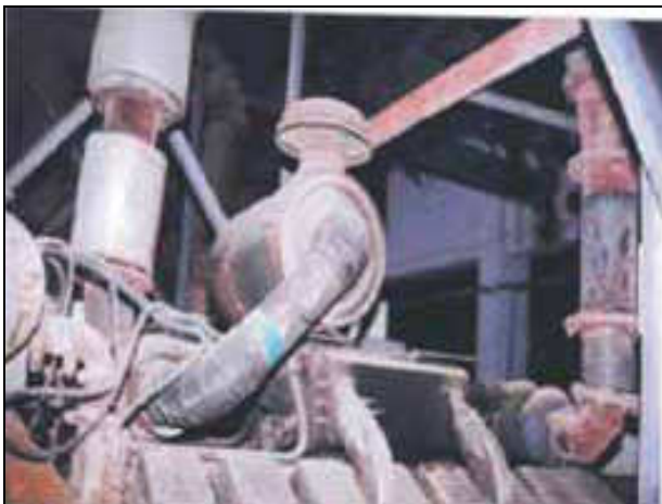
DG set with conventional dry type air filter
