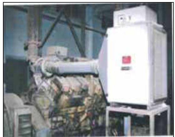
Air intake retrofitted with Electrostatic Air Filter
