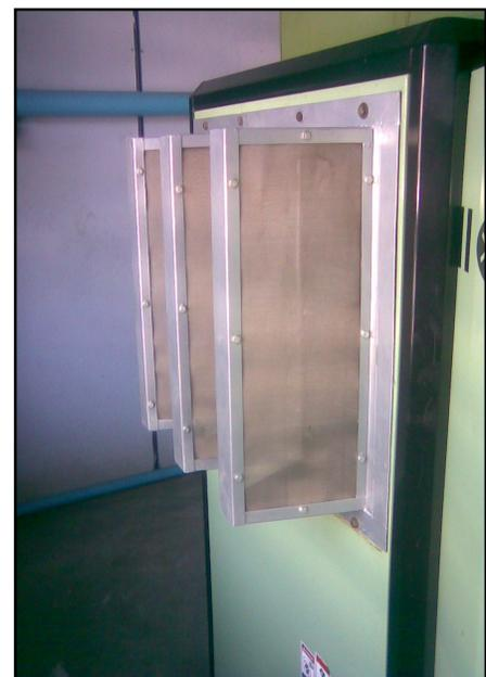
Courtesy:- BOJE compressor manual / Compressor hood V type pre-filter reduces ambient dust.
