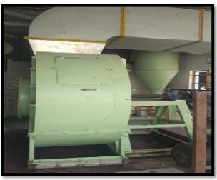
I Image – Routine Thermal Imaging of motor is easy now and quick to target & reduce Hot Spots. II Image – Waste collection Suction centrifugal blower rating 55 KW, 75000 CFM flow @ 2200 Pascal.
