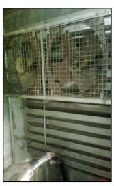
Courtesy:- Cummins DG Manual /Cross ventilated DG engine/ Forced Fresh air at air inlet.
