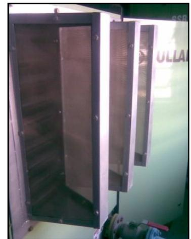
As well to prevent this to happen, the user can think of doubled area V shape filter as pre-filter outside the existing fins on the outer cover of the outdoor unit. The user by this, can prolong the choking of the condenser fins from outside, thro out the season. The user can clean the pre-filter once in a week or month suitably.
